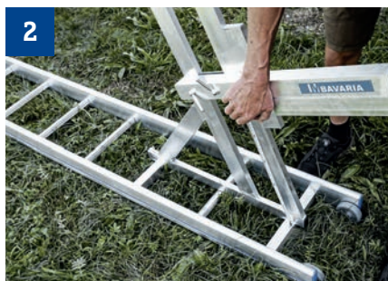
2 Adjust the position of the posts to match the roof overhang.
