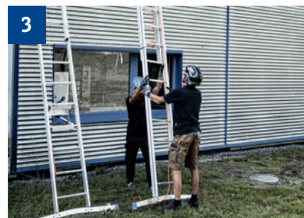
3 Erect the ladders.
