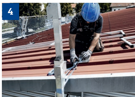
4 Anchor the posts with lashing straps.
