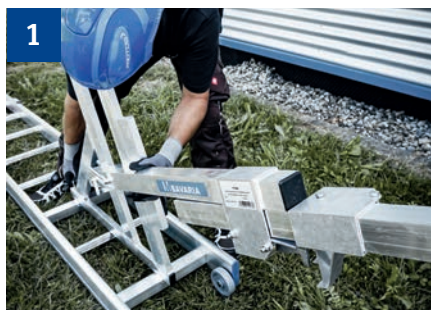
1 Attach the guardrail posts to the ladders.
