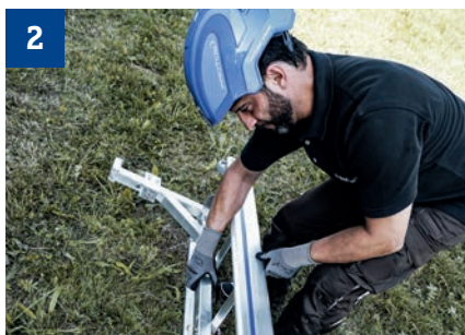
2 Attach the railing posts to the ladders.
