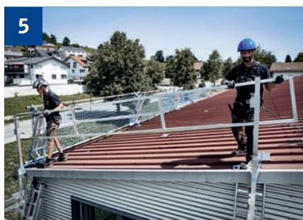
5 Hook the rail frames into the posts.
