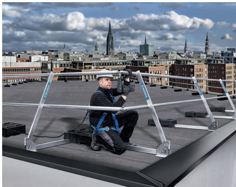
NEO 40 N assembly example with inclined post
