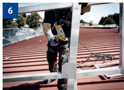
6 Secure the guardrail by the wedge locks.
