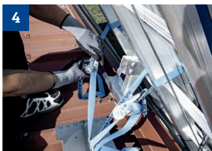
4 Anchor the ladders with lashing straps.
